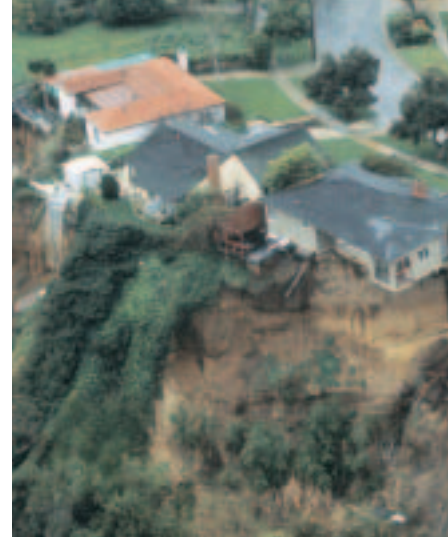
Figure 4.3 In Malibu, California, heavy winter rains during 1983 caused landslides on steep, unstable slopes. As a result, several homes suffered serious structural damage.
