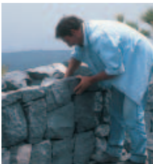
Figure 3.10 Landscape architects often use this “mass” method of joining to design stone retaining walls and split-rail fences.
