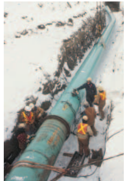
Figure 2.17b) Workers installing a gas pipeline
