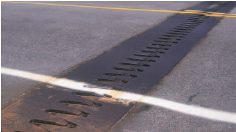
Figure 2.17a) When temperatures are low the space between metal joints is large. When temperatures rise the space between the metal joints closes up.
