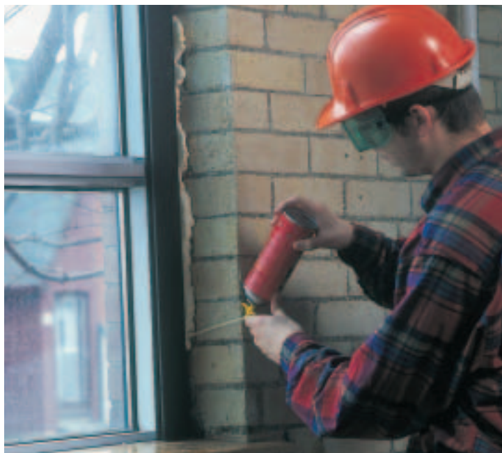
Figure 2.2 A foam is a colloid of a gas in a liquid. The foam in this photo is used for insulation. It comes out of the can as a fluid, and then hardens in place to seal cracks.
